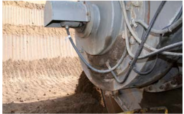
Anbaustelle am Schaufelrad / Mounting position at the bucket wheel
